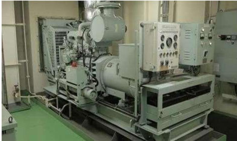
**Gambar 2. 1 Diesel Generator**
