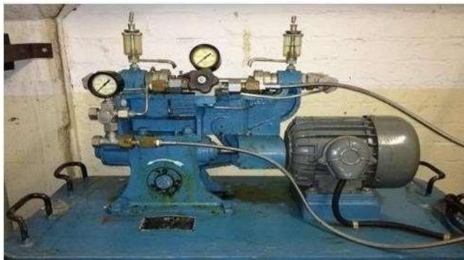
**Gambar 2. 6** Electro Motor Pada Booster Pump
