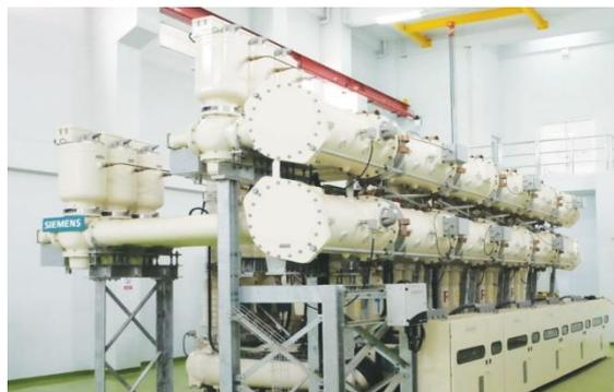
Gambar 2.18 *Gas Insulated Substation*
