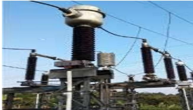
Gambar 2.14 Transformator Arus
