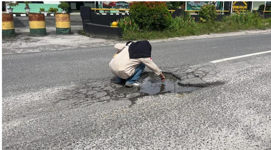
Gambar 3.9 Lubang (Hasil Survey dilapangan)
