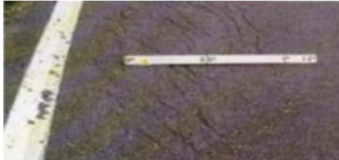
Gambar 2.21: Patah slip (Lestari, 2020)
