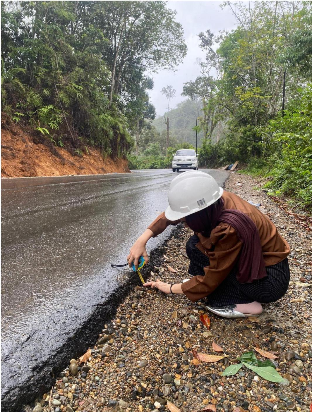
Gambar L.3: Mengukur Tebal Perkerasan Jalan
