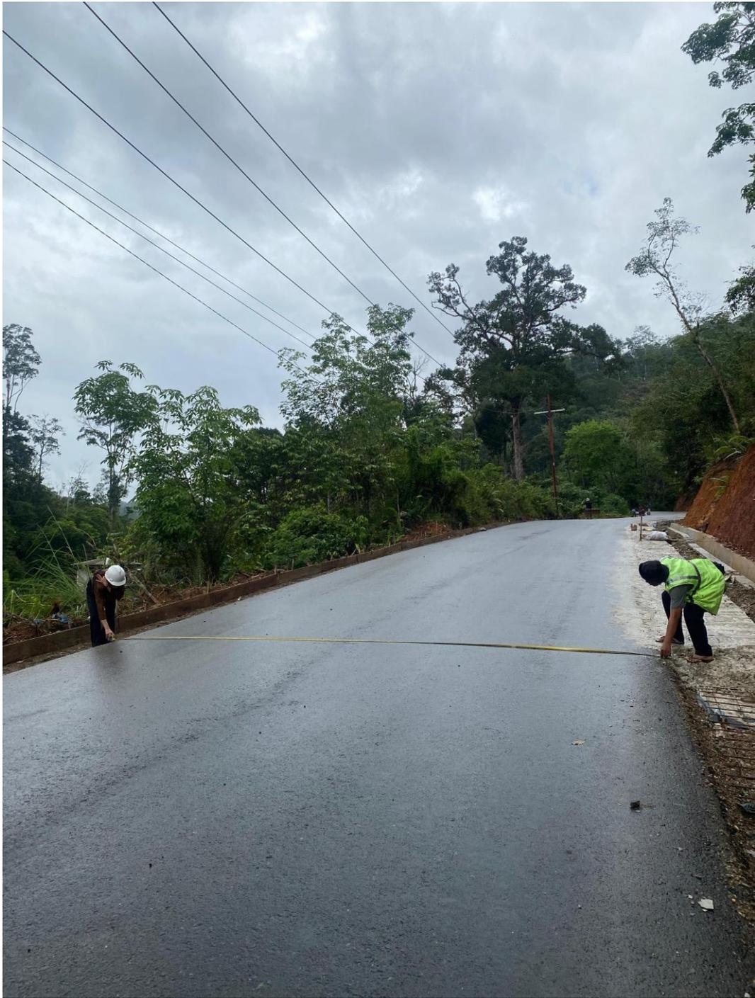
Gambar L.2: Mengukur Lebar Jalan
