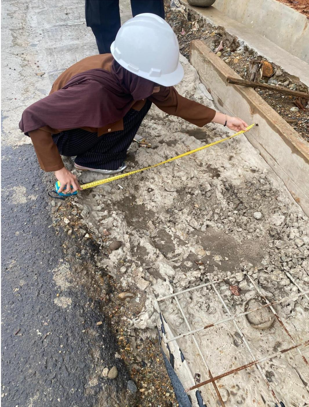
Gambar L.4: Mengukur Bahu Jalan
