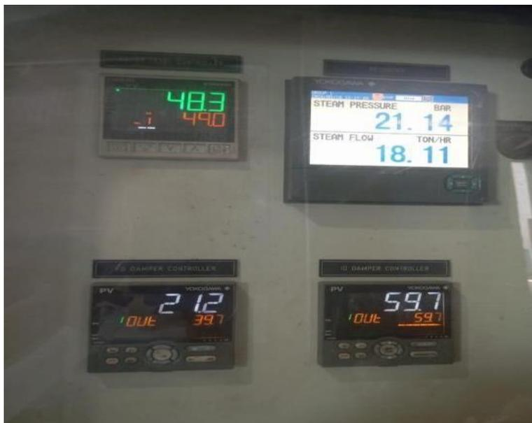
Gambar 3. 5 Control Panel boiler
