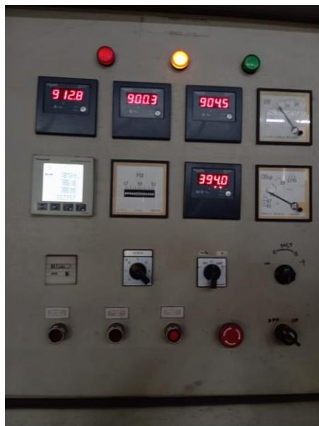
Gambar 3.2 *Control Panel Turbine*
