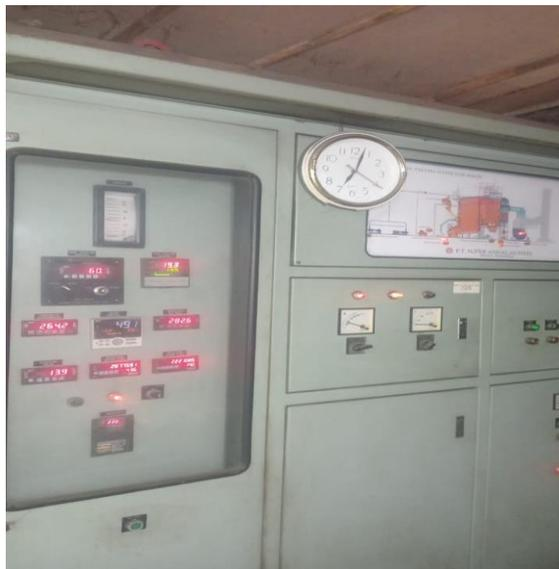
Gambar 3.6 Panel Parameter boiler
