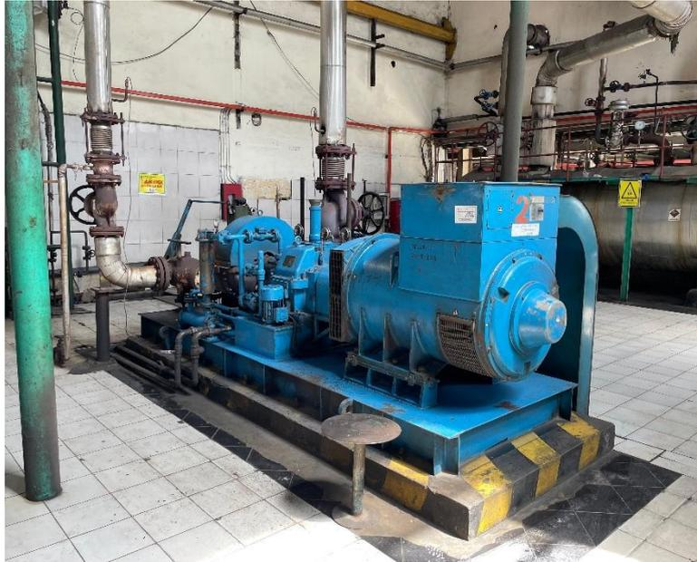
Lampiran Gambar 3: Generator Turbin 800 kW
