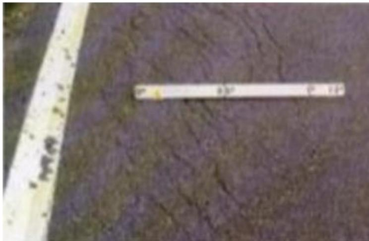
Gambar 2.21 Patah Slip (Lestari, 2020).
