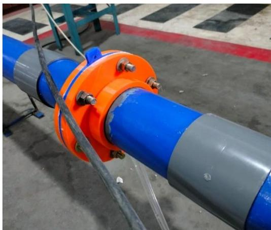
Gambar 4.7 Sambungan Pipa Yang Telah Dipasang
