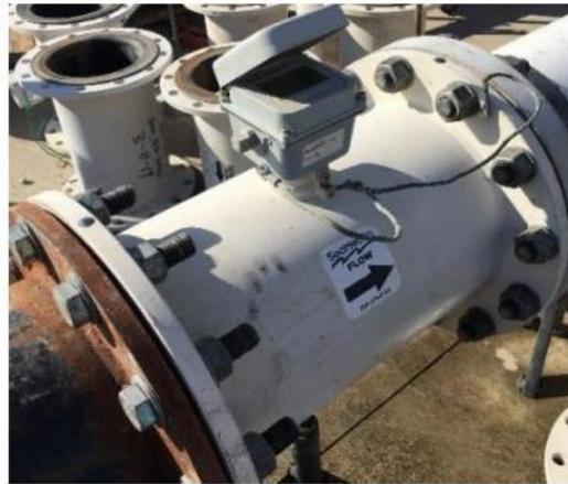
Gambar 2.17 *Magnetic Flowmeter* (Styles et al., 2020)
