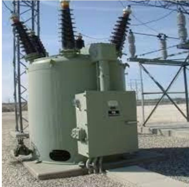
Gambar 2. 2 PMT 250 KV (Irwan. 2019)
