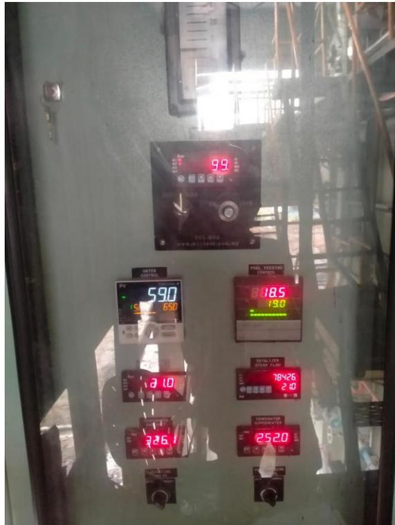
Gambar 3.8 Panel Parameter boiler
