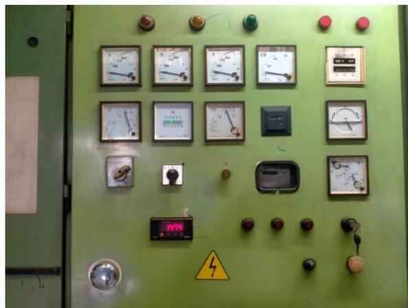
Gambar 3.3 Control Panel Turbine
