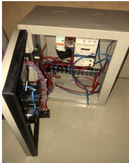
Gambar 4. 13. Wiring Pengontrol Conveyor otomatis
