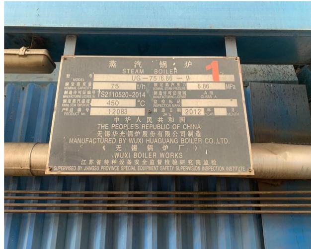
Gambar 2.2 Name Plate Boiler
