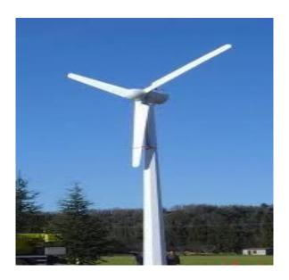
Gambar 2.1 Turbin Angin Sumbu Horizontal
