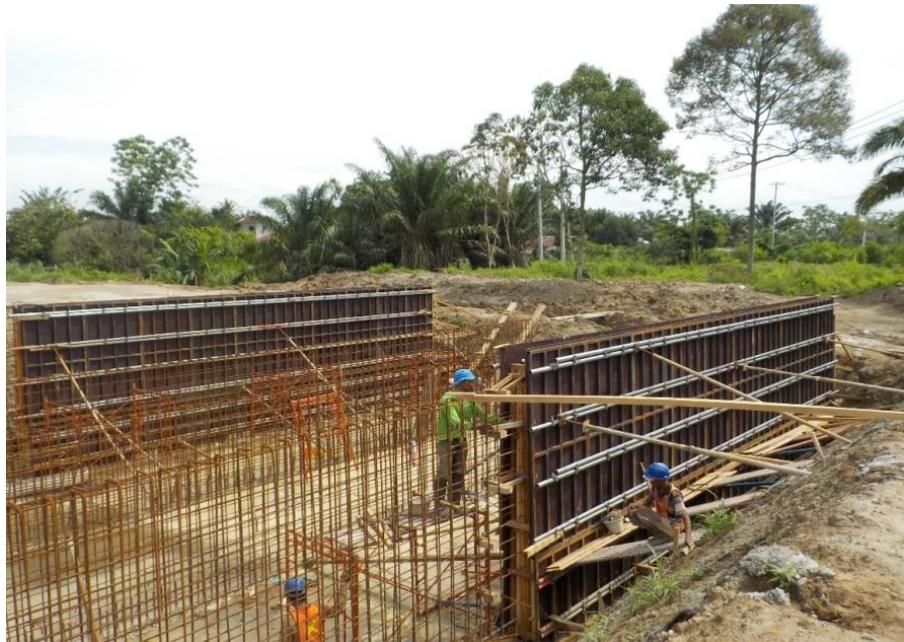
Gambar L4.4: Pemasangan Bekisting Dinding Samping Kanan Kantung Lumpur Kanan
