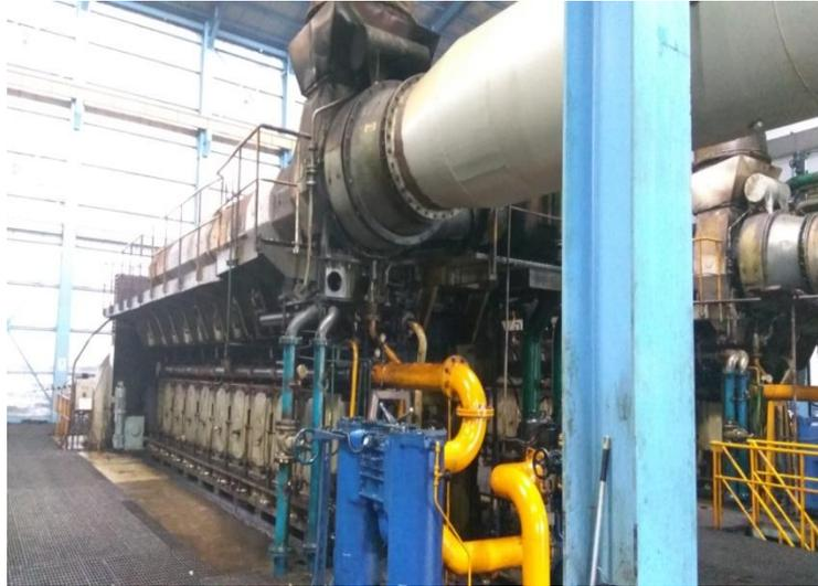
Gambar 3.1. motor diesel
