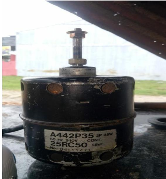
Gambar 3.16 Motor *Fan Indoor Ac*
