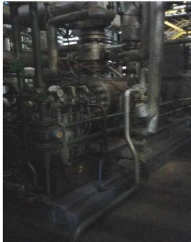
**Gbr 4.2. Pompa air umpan ketel uap (Boiler Feed Pump)**
