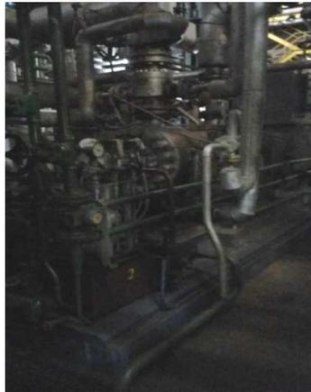
Gambar 2.5. Pompa air umpan boiler
