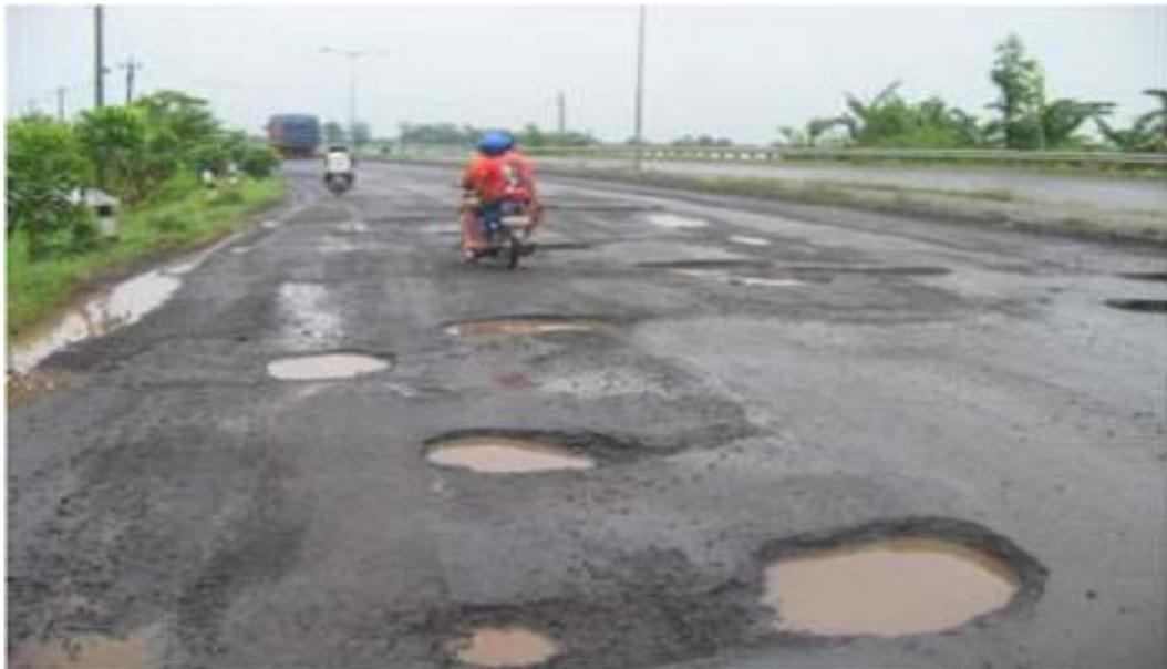
Gambar 2.11: Lubang (Bina Marga, 1983).
